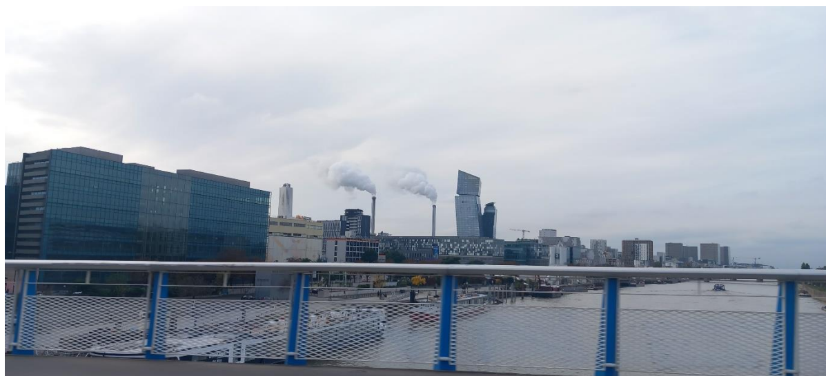
Figure 1: View of the incinerator Ivry-Paris XIII
